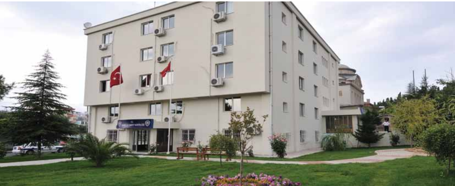
Pendik District Police Headquarter (Retrofitting Completed)
