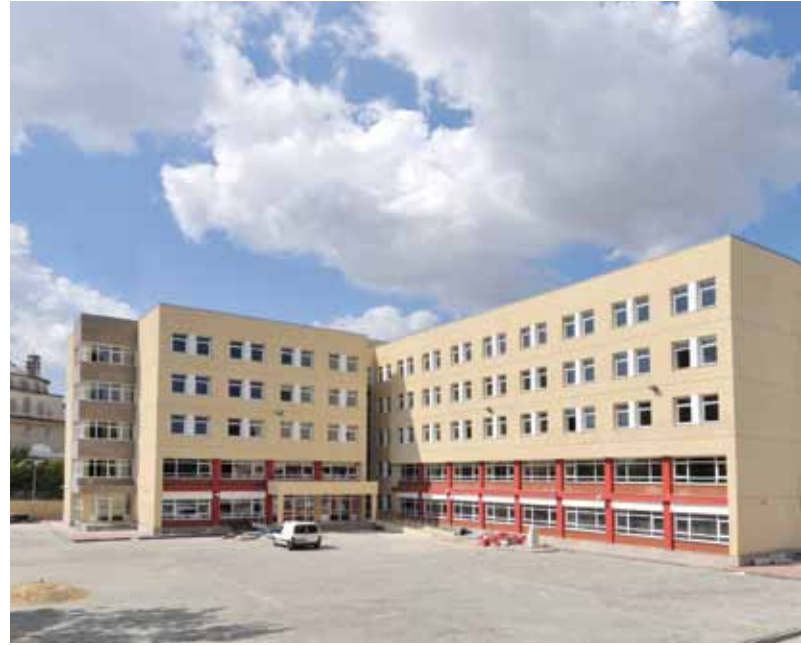
Energy Efficient Smart School, Bahçelievler Kazım Karabekir Primary School
