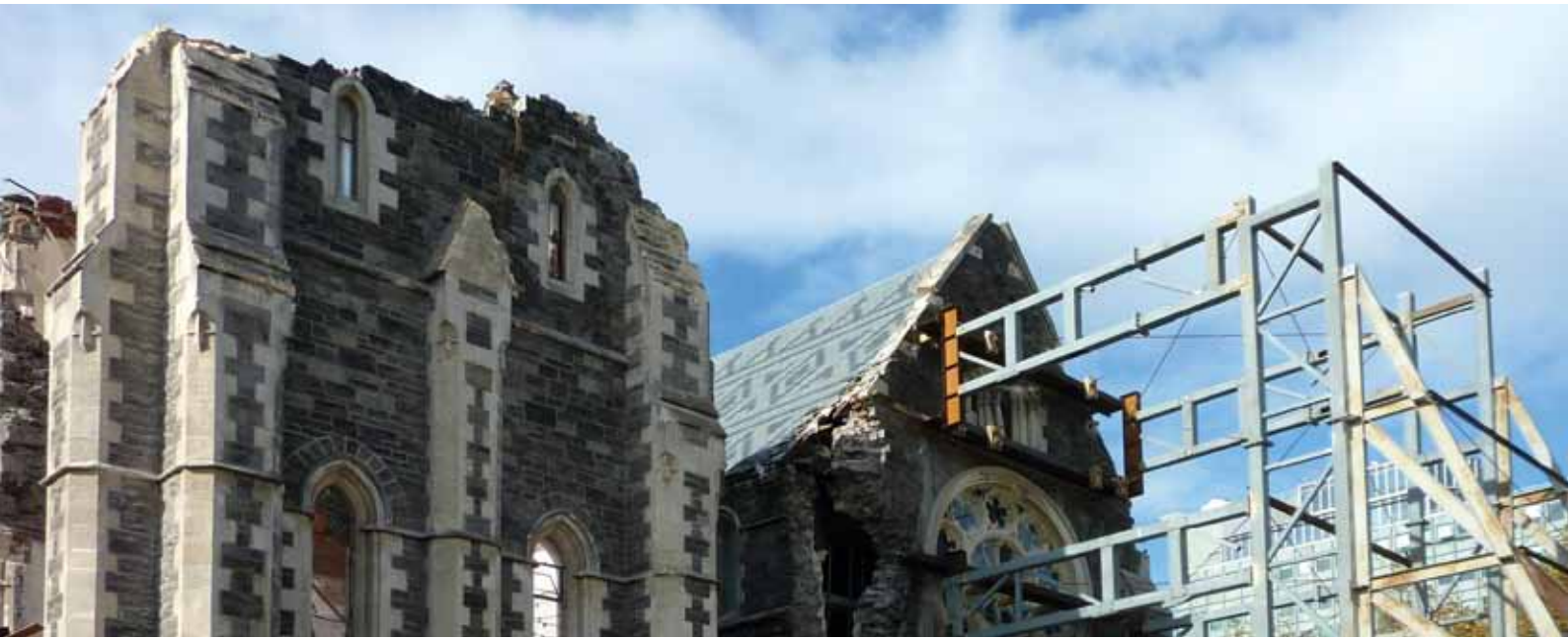
An Example of Retrofitting Work on Historical Buildings, ChristChurch Cathedral, New Zealand
