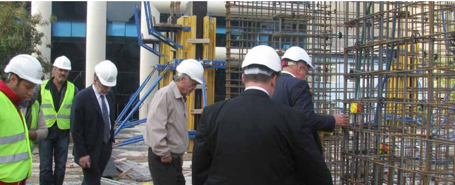
Reconstruction Site Visit
