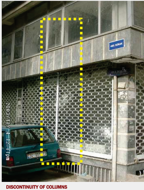
FIGURE 12 INAPPROPRIATE MODIFICATIONS ON BUILDING
