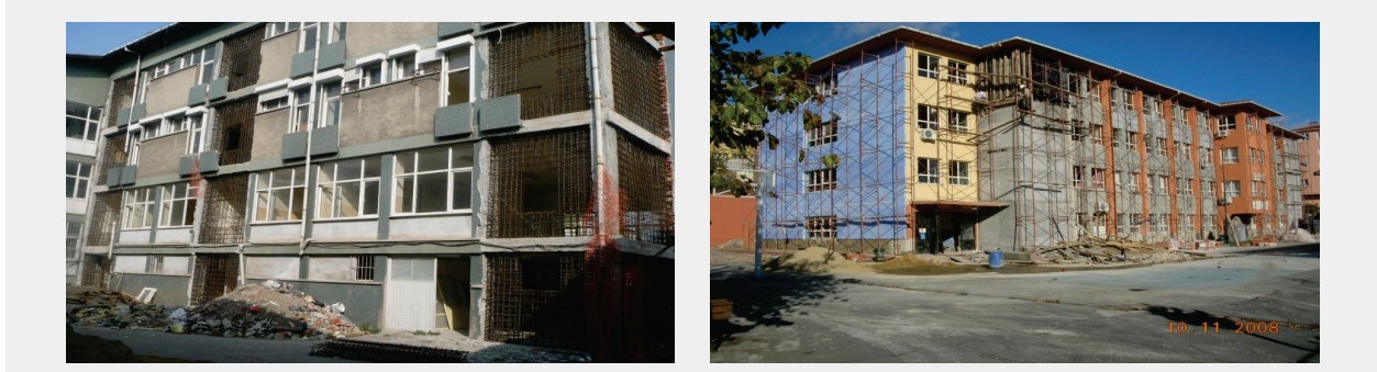
FIGURE 19 BUILDING RETROFITTING ACTIVITIES
