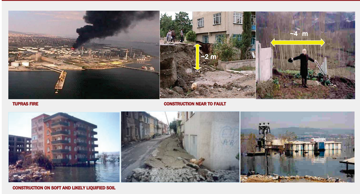
FIGURE 16 BUILDINGS NOT IN CONFORMITY WITH SOIL CONDITIONS
