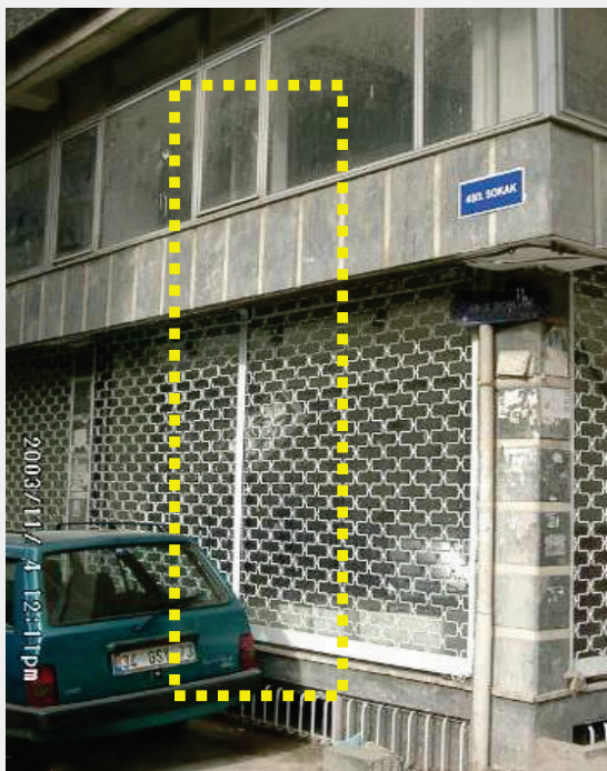
DISCONTINUITY OF COLUMNS
