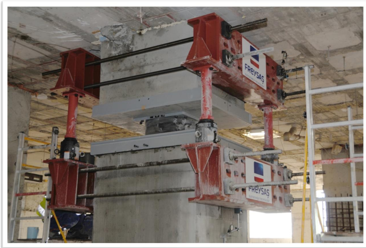
Marmara University Prof. Dr. Asaf Ataseven Hospital – Seismic Isolators
