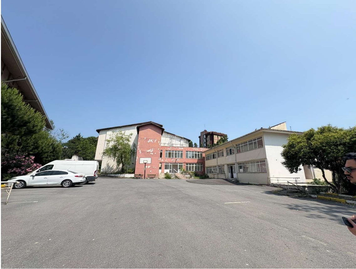
Photos 1: Project Area
