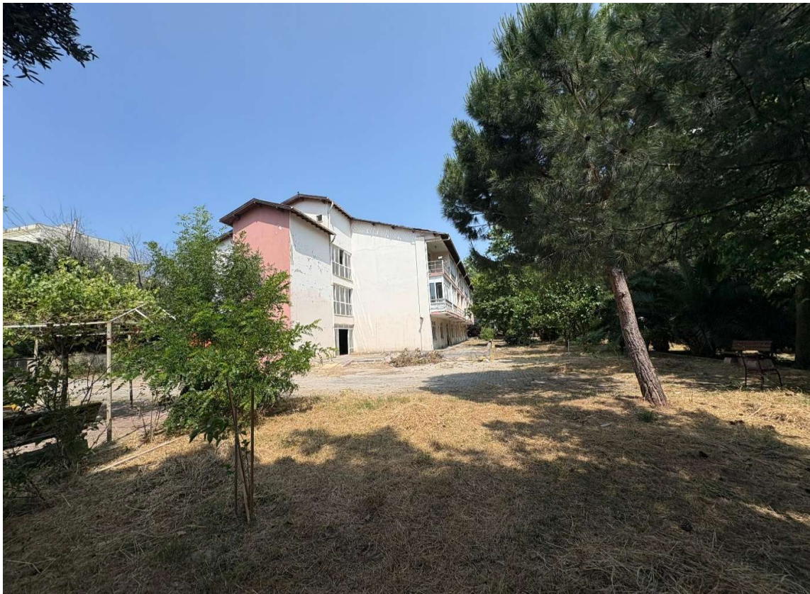
Photos 2-3: Project Area
