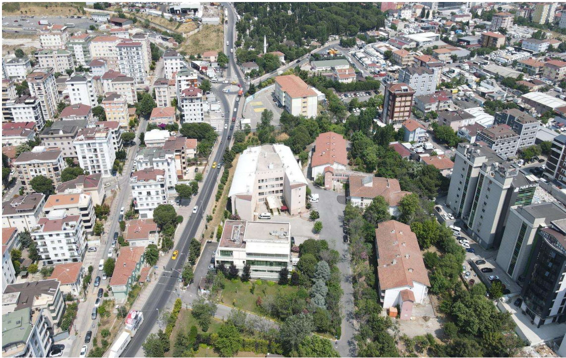
Photo 12-13: Drone Photos / Project Area
