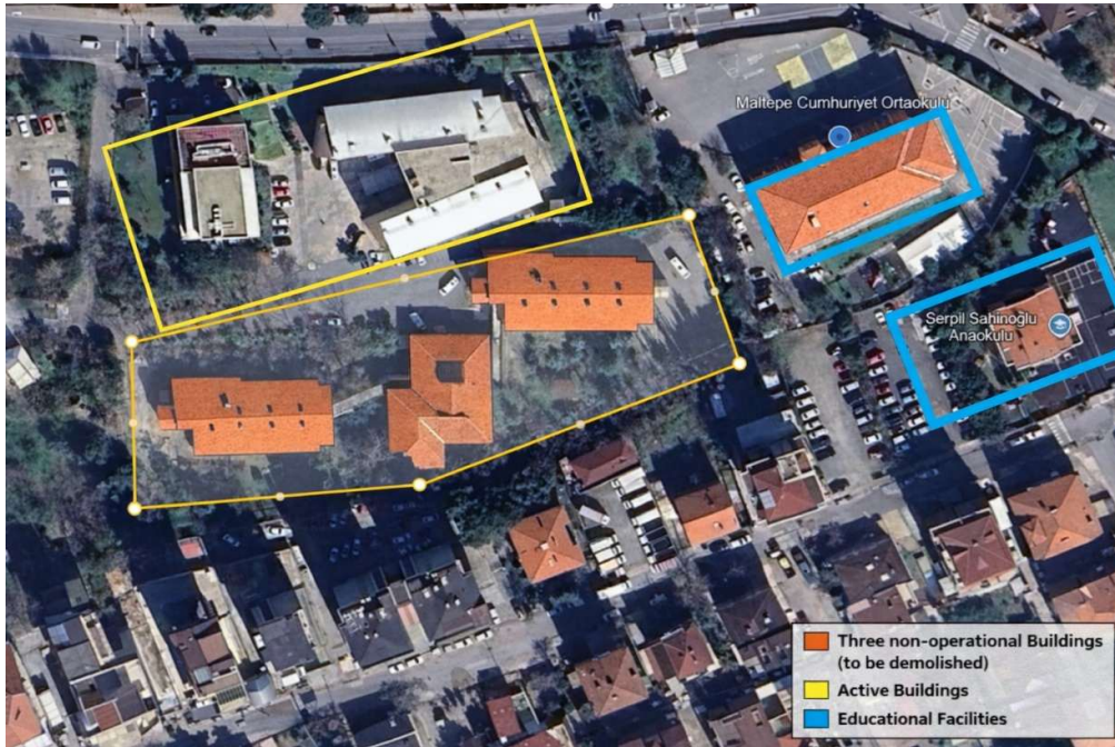
Figure 1: General View of Maltepe Nursing Home Project Site (Maltepe, Istanbul)
