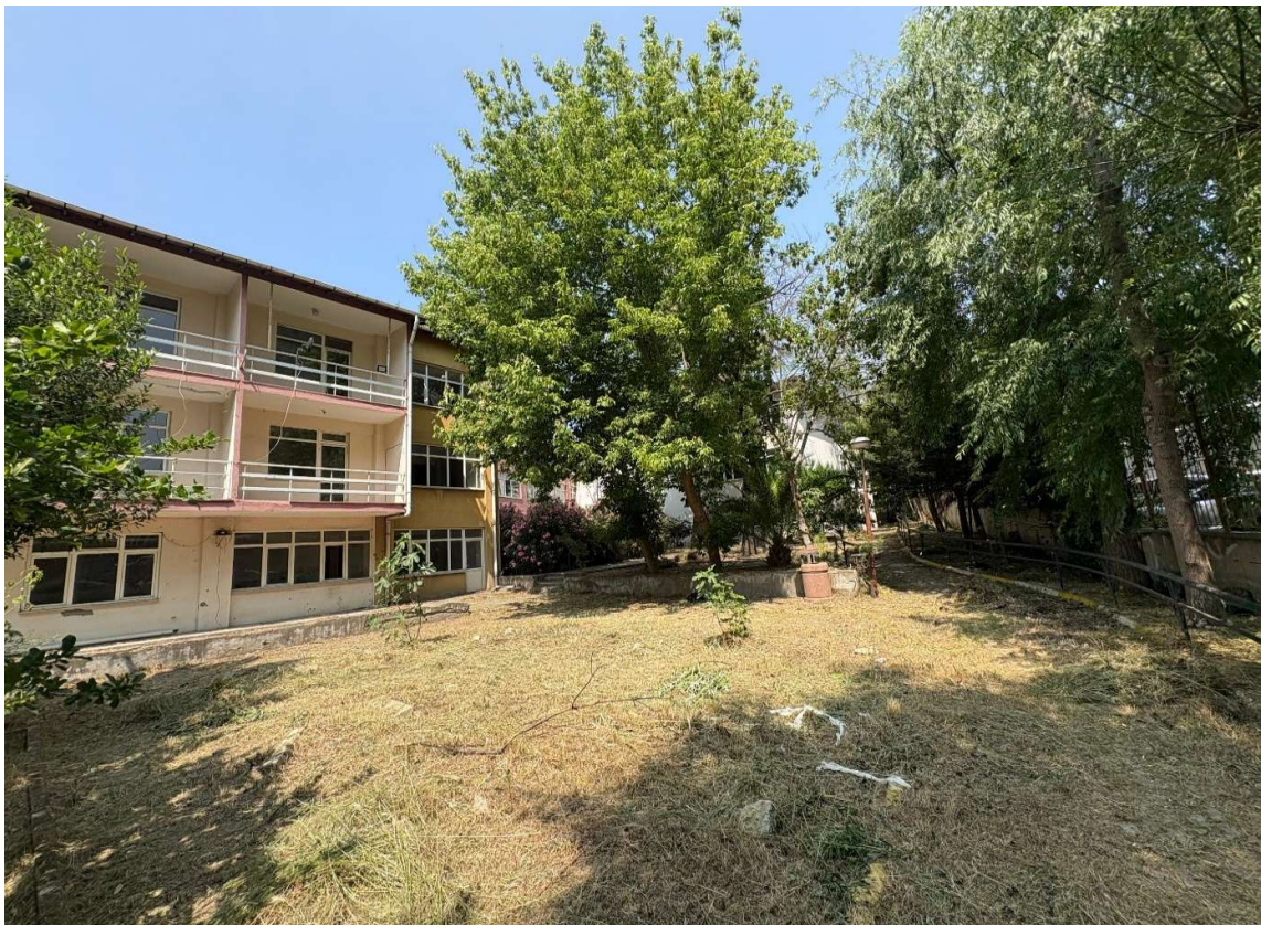
Photos 4-5: Project Area
