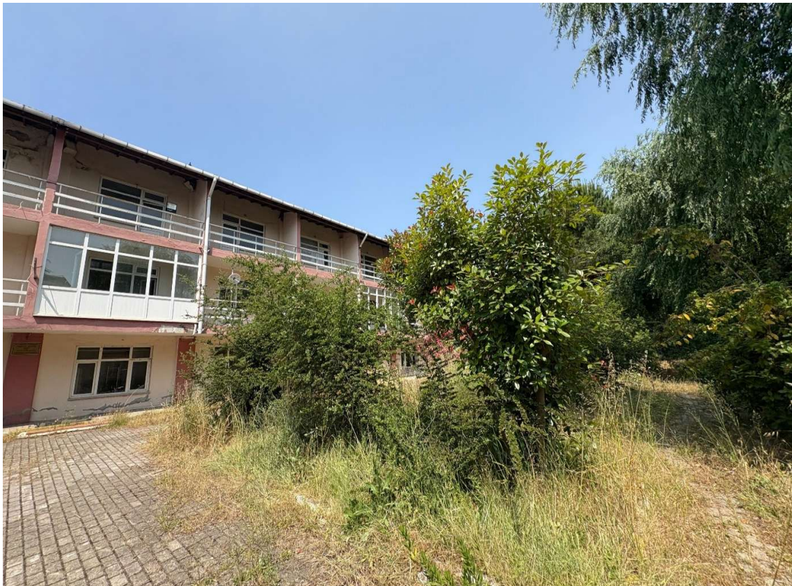
Photos 6-7: Project Area
