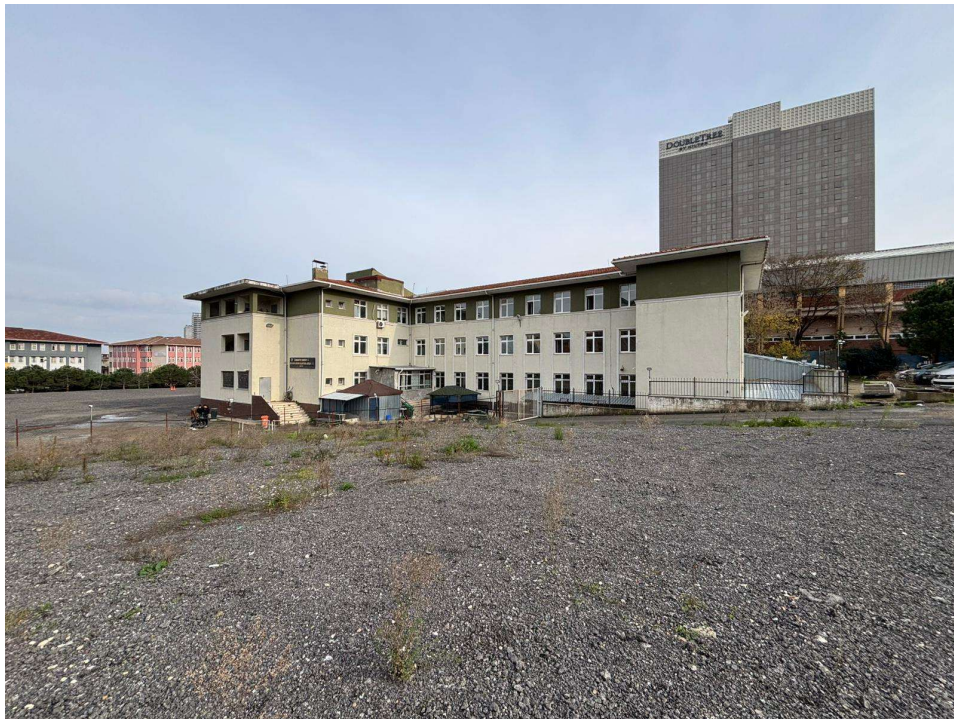
Photo 2: Electrical Workshop Building
