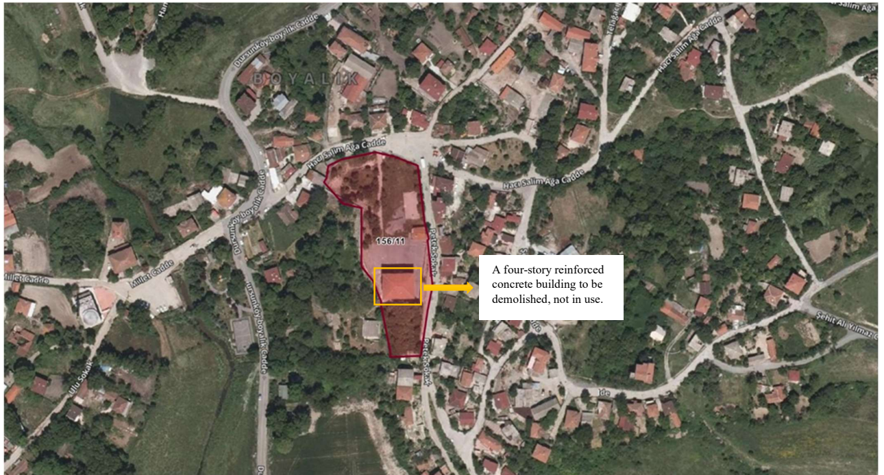
Figure 1: General View of Arnavutköy Boyalık Primary and Secondary School (Arnavutköy, Istanbul)
