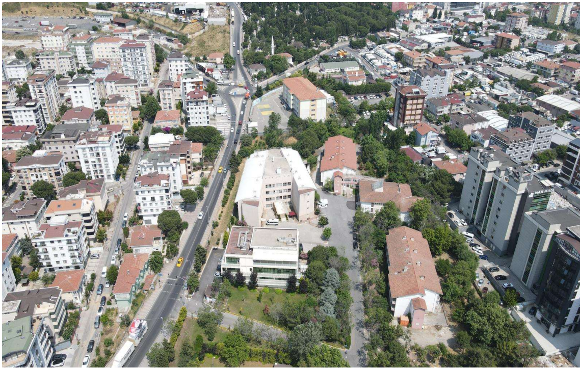
Photo 12-13: Drone Photos / Project Area
