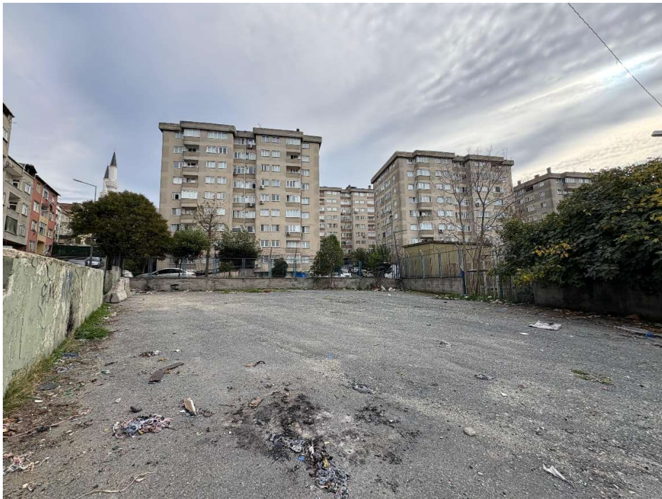
Photos 3-4: Project Area
