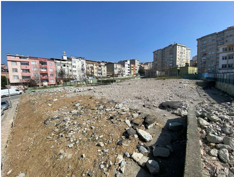
Photos 5-6: Project Area
