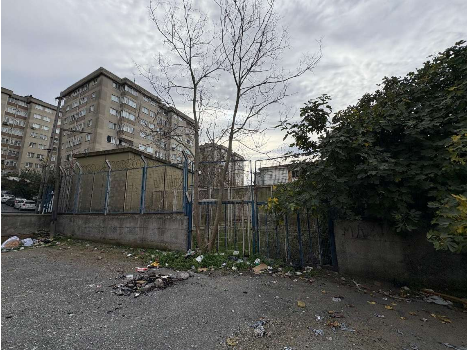
Photos 11: Project Surrounding Area / Transformer
