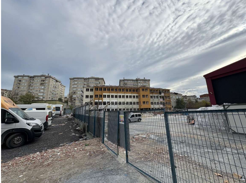
Photos 9-10: Project Surrounding Area
