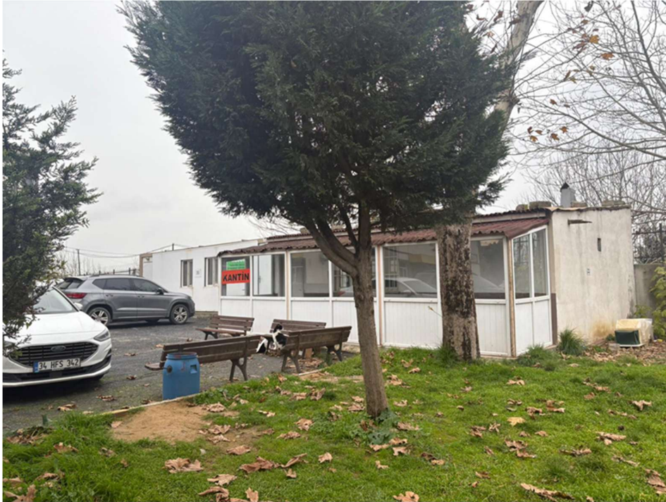
Photo 10: Project Area and Other Structures (Canteen)
