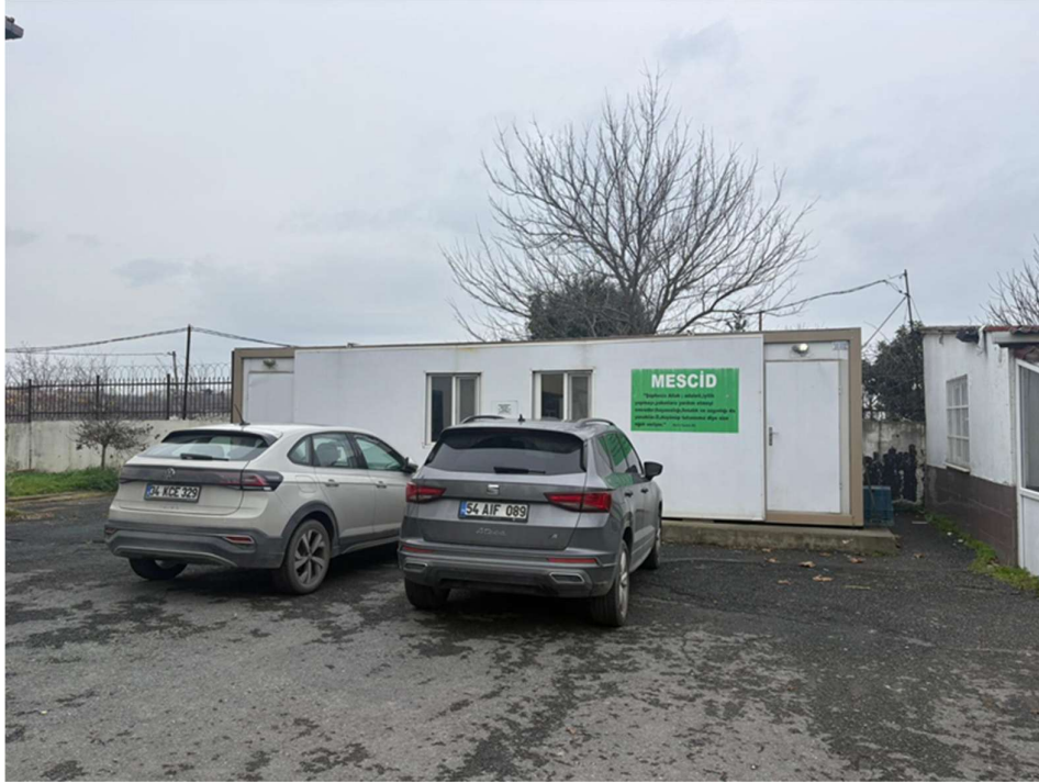
Photo 11: Project Area and Other Structures (Prayer Room)
