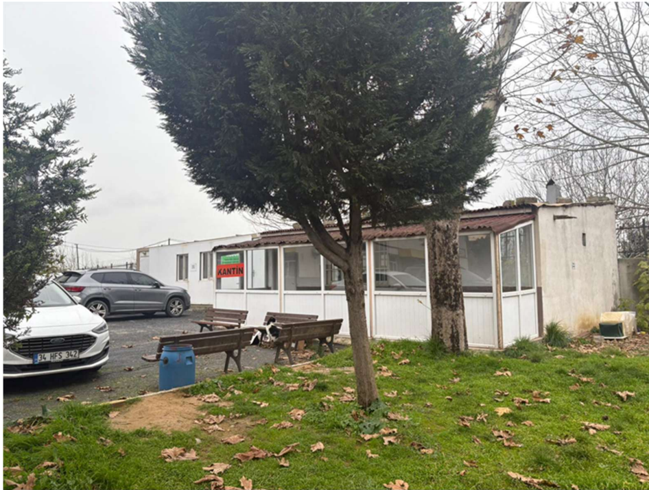
Photo 10: Project Area and Other Structures (Canteen)
