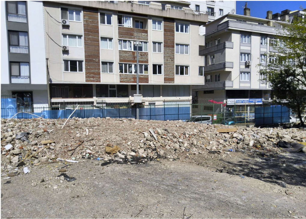
Photo 8,9,10: Site Area of Former Staff Housing Buildings (Demolished)
