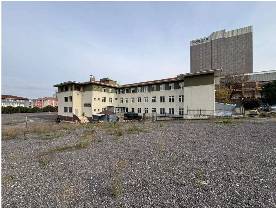
Photo 2: Electrical Workshop Building
