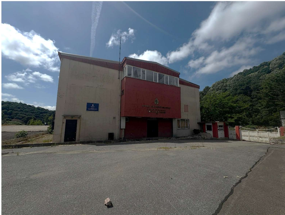
Photo 8-9: Project Area and Other Structure – Gymnasium (outside the subproject scope and to be retained)
